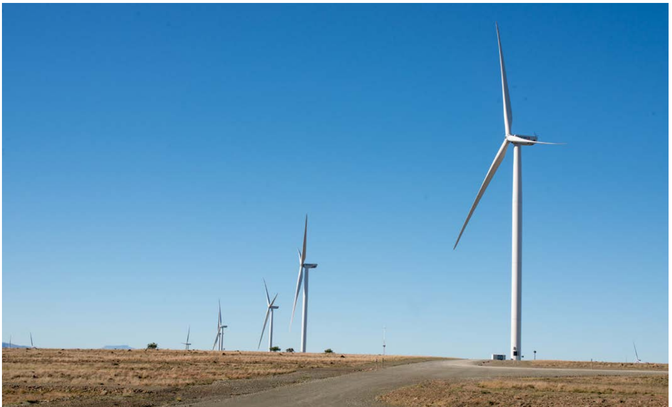
Cennergi's Amakhala Emoyeni windfarm
