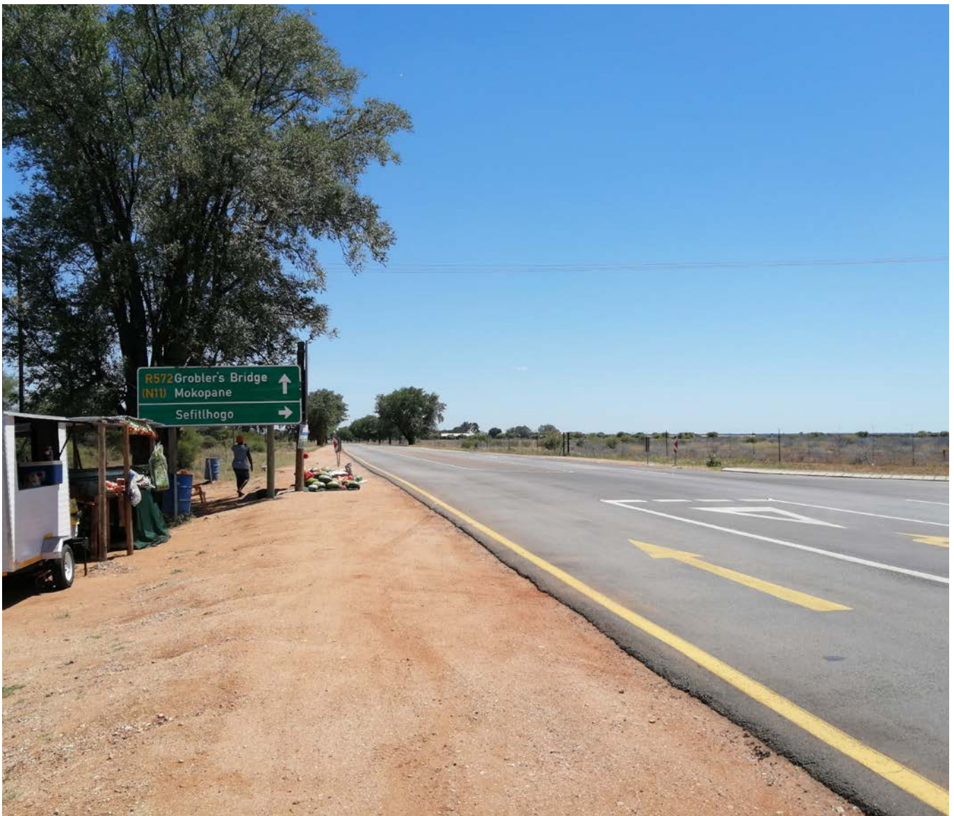
Road upgrade at Ga-Seleka in Limpopo
